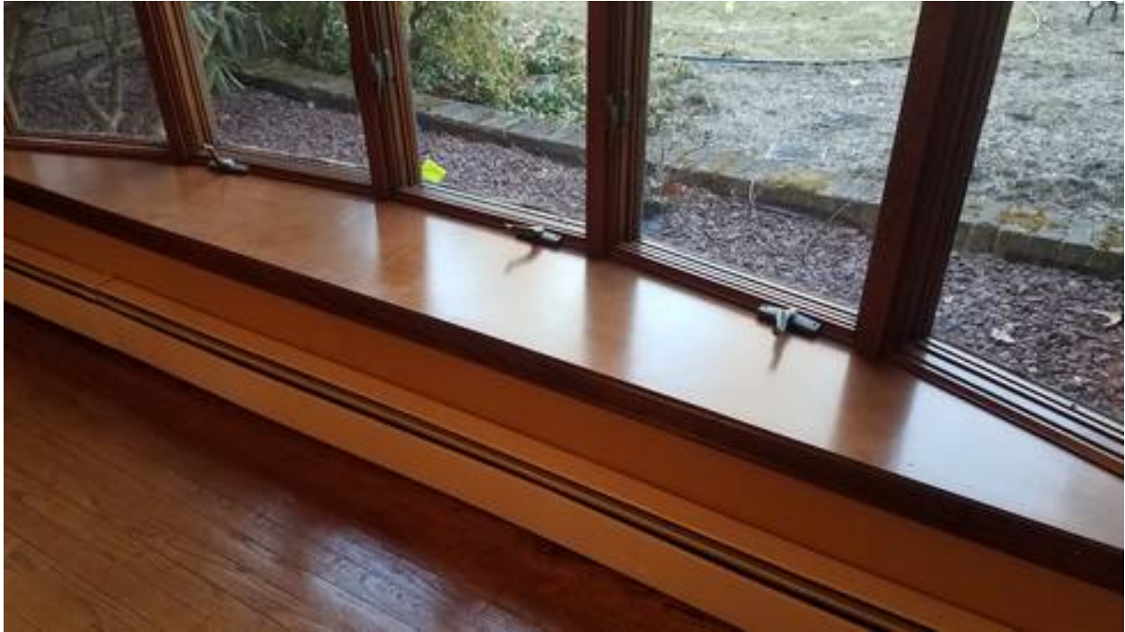
7C.17 Stuck/binding original, wooden, casement windows. Repair is recommended as needed here and there
