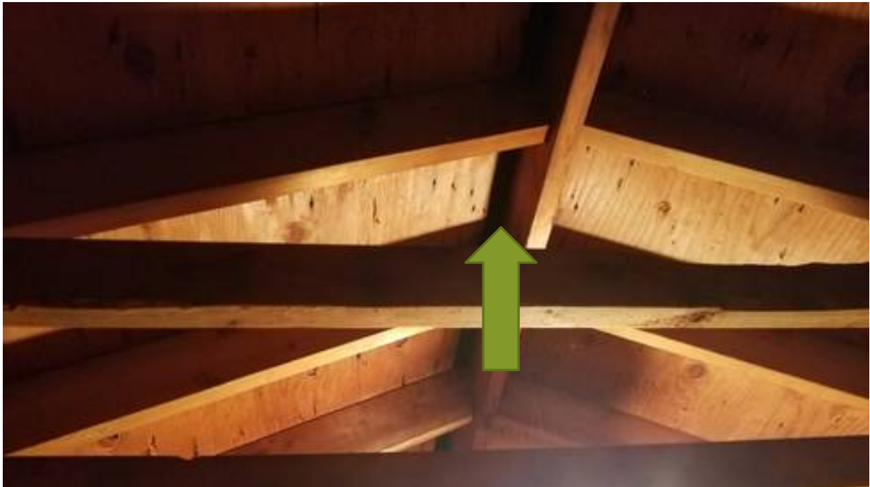
1C.03 Condensation/excess humidity/indoor air quality concerns: Typical humidifier found; moisture meter indicates excessive moisture; mold-like substance seen; peeling exterior paint; rot; stains visible in basement and in exterior walls
