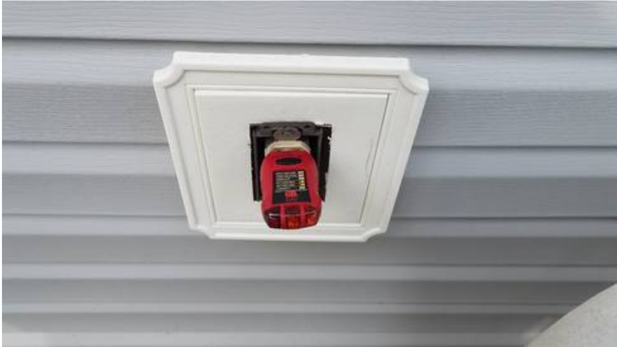
5C.64 Receptacles: painted many areas. This is a safety and function concern. Recommendation: Replace
