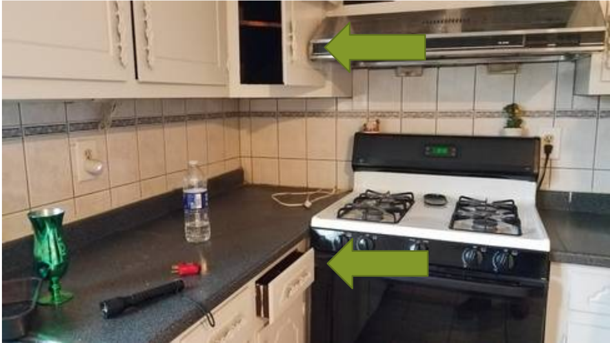
9E.20 Insulation comparative rating: fair-r-13-19 Filters and hood grease laden for kitchen exhaust fan. Recommendation: Replace for function and safety
