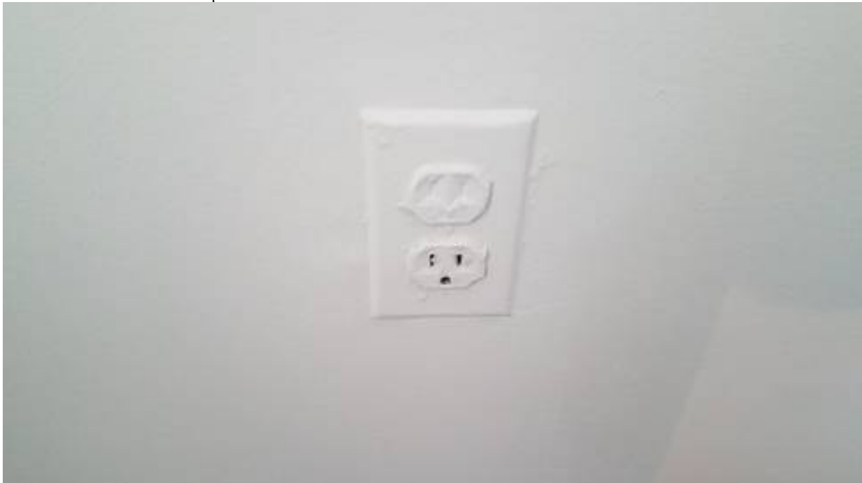
5A.40 Electrical comparative rating: apparently poor
