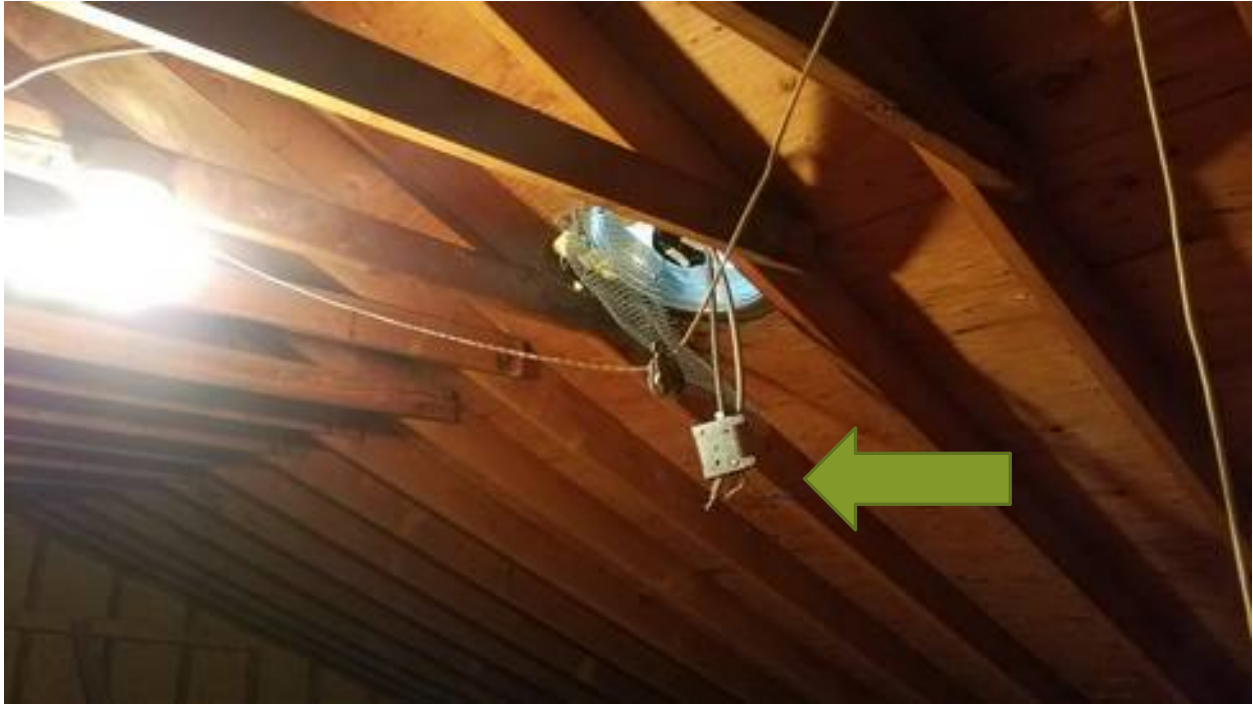
3C.33 Vent, ridge: Missing. Repair is recommended and add soffit ventilation as well for proper function
